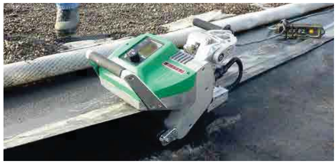
The GEOSTAR easily welds 240 m without difficulty in a single pass during a field test (South Africa)..
