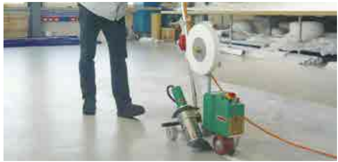
Welding tape at maximum speed.
