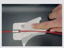
**Step 3:**Removing the excess welding rod with Quarter Moon Knife or Trimming knife.
