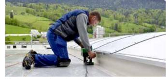
Whether on or at the roof parapet or welding domed skylights, connections, or small terraces – the UNIDRIVE 500 shows its worth when space is tight.
