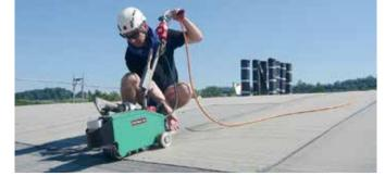
Flameless welding of modified bitumen with the BITUMAT. B2.
